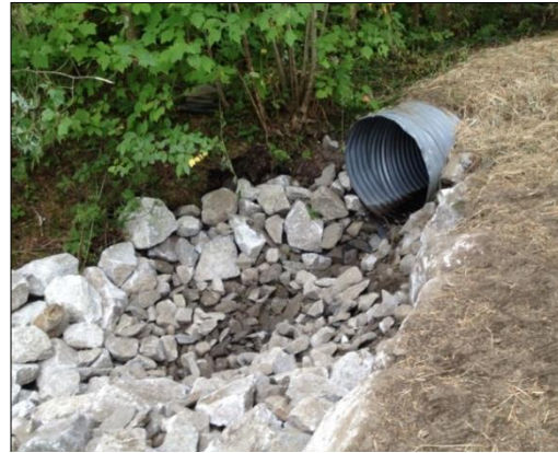
AFTER – Stone-lined settling pool and outfall below culvert, allowing sediment to settle out before discharging into Lake Seymour. . Photo credit: M. Stickney, VTDEC
