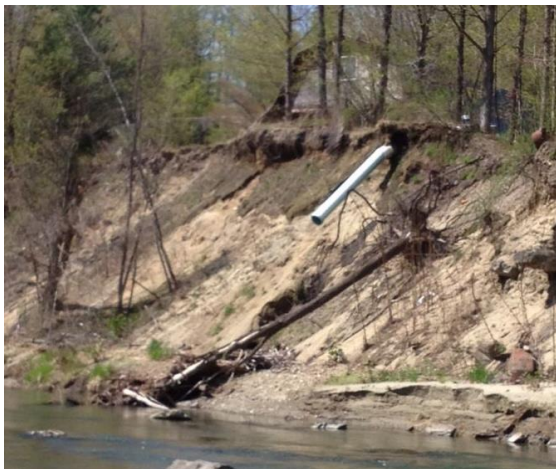
Stormwater outfall contributing to bank failure. Photo credit: J. Pease, VTDEC
