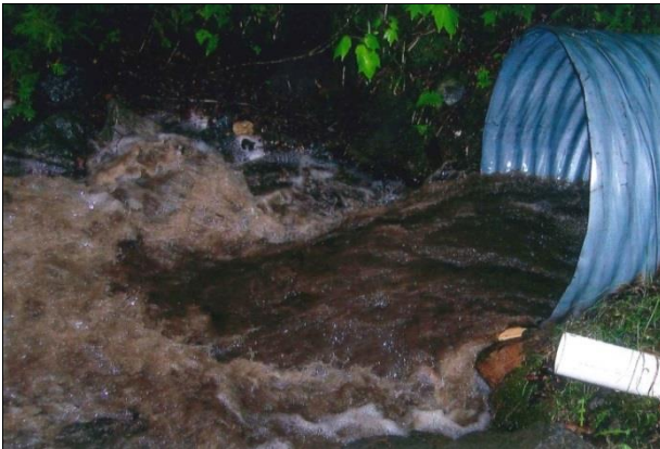
BEFORE – Sediment-laden water discharging to Lake Seymour. Photo credit: V. Bushee
