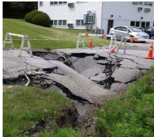
Road damage from stormwater runoff. Photo credit: J. Pease, VTDEC
