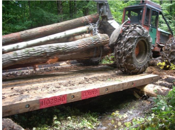
Skidder Bridge, Photo Courtesy of the VT Department of Forests, Parks and Recreation
